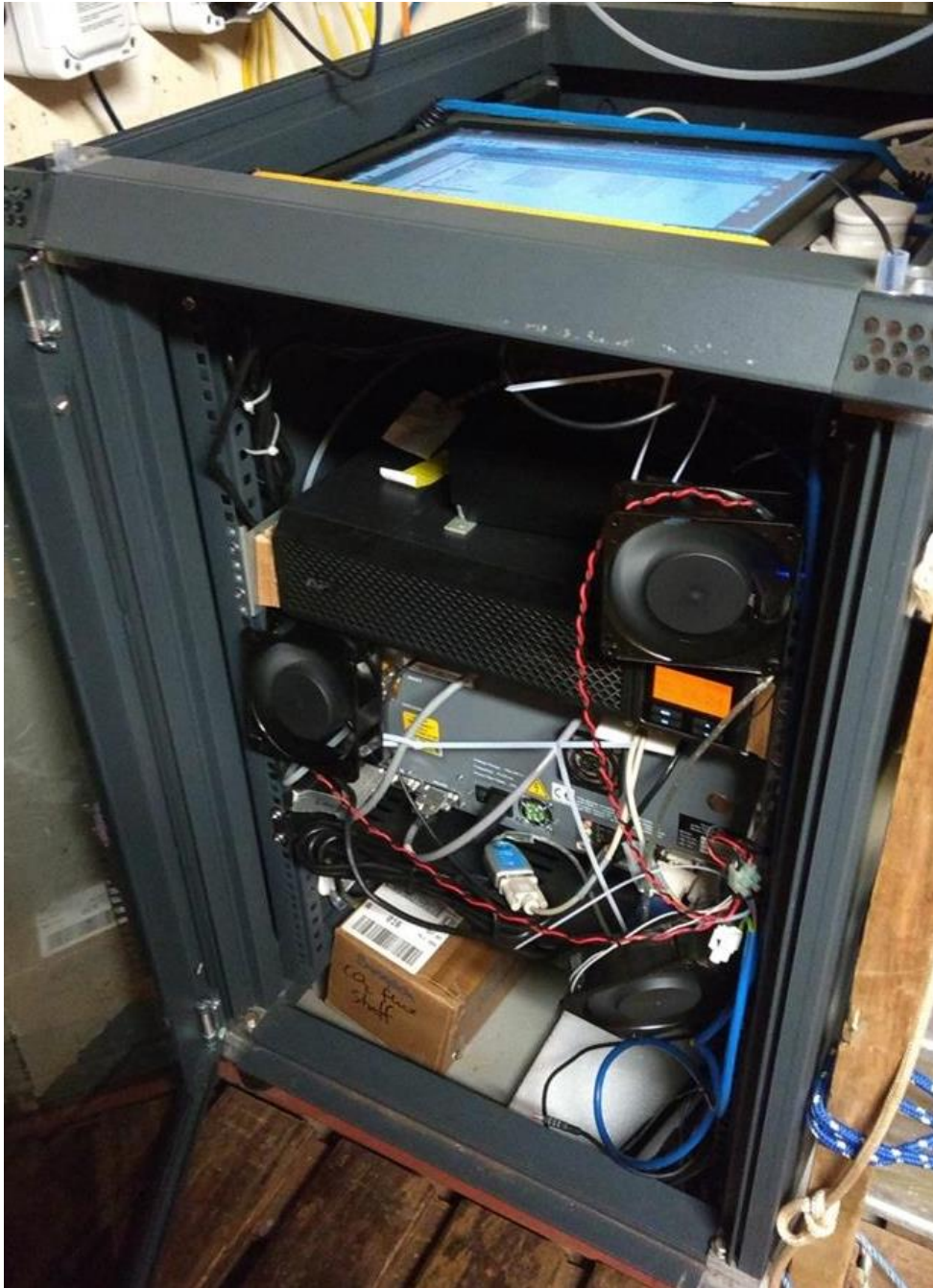
Figure 22:- Installation of additional fans to assist cooling of mail room Picarro
