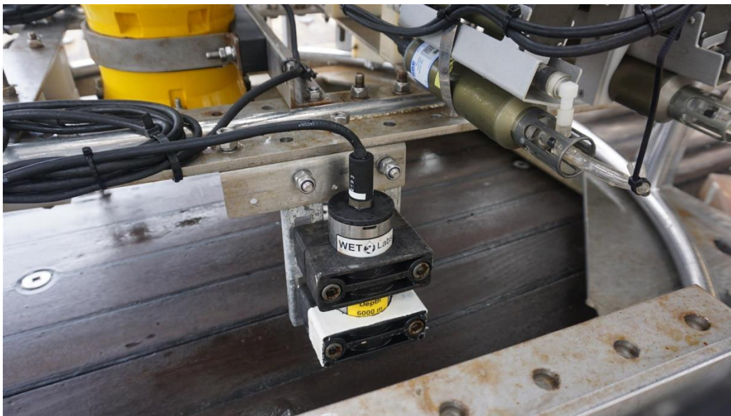
Figure 19:- Seabird Eco-FLBB installation
